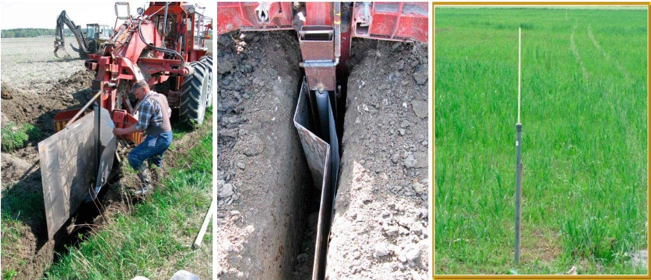
Fig. 3. Machinery for installing the plastic sheet (left and middle pictures) and a groundwater pipe with a “floating antenna” to show the groundwater level (right picture).
