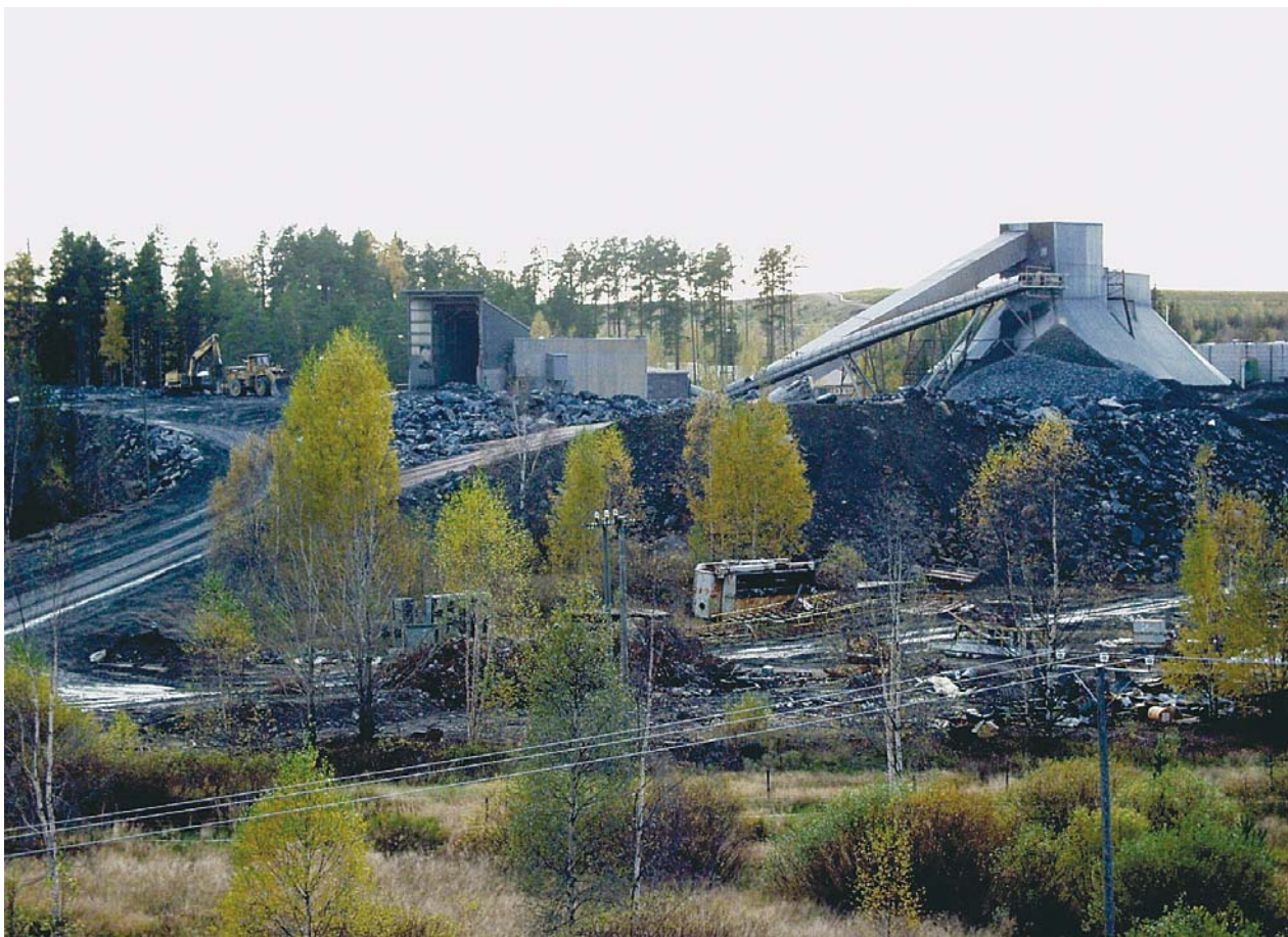
Figure 41. The mine site contains a number of specialized buildings and structures, such as the crushing mill shown here, at the Hitura Ni mine, Nivala, Finland. In general, such infrastructure is dismantled during mine decommissioning and closure, if they cannot be used for other purposes or for processing ore from nearby deposits.
