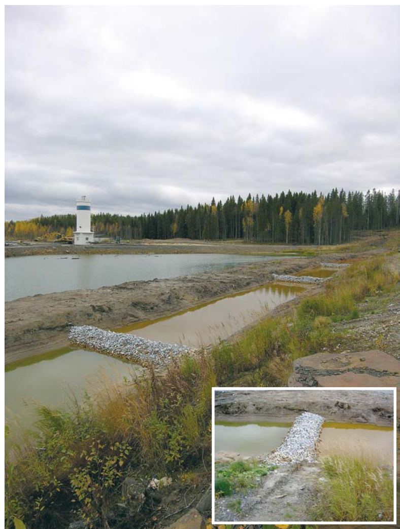
Figure 17. BAT for treating acid mine drainage includes neutralizing with lime. The Lahnaslampi talc mine in Sotkamo has a series of limestone batteries to filter the water discharged from the waste rock disposal areas.
