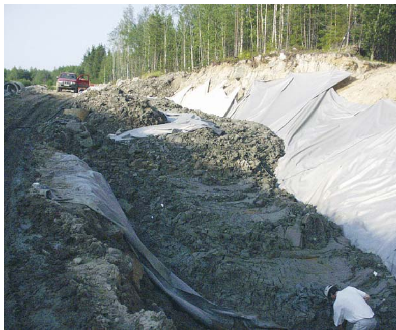
Figure 40. If a tailings impoundment is constructed over a permeable substrate, there is an enhanced potential for groundwater contamination. Site remediation measures may include arresting discharge of water from the impoundment by addition of impermeable compacted materials in various ways. The example shown here involves the use of compacted clay directly overlying bedrock. The location of tailings impoundments should only be decided after thorough characterization of soil structure, with areas underlain by coarse, poorly consolidated materials to be avoided.
