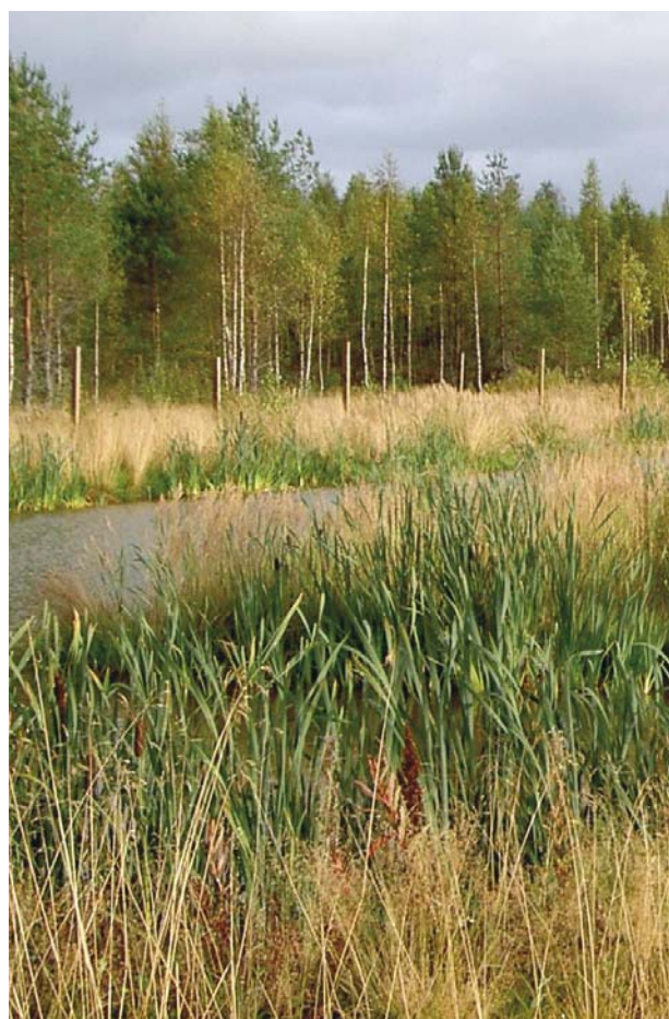
Figure 43. Aerobic wetlands are highly suited to treatment of near-neutral ( pH > 5 ) waters containing elevated Fe and Mn. Precipitation of Fe and Mn compounds reduces trace metal abundances in the water, while vegetation modulates flow rates and promotes retention of precipitates within the confines of the wetland basin (Hammalahti Cu-Zn mine, Pyhäselkä, Finland).
