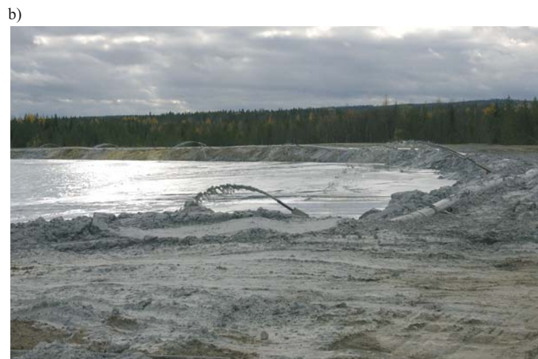
Figure 3. a) Waste rock pile at Siilinjärvi apatite mine, Finland, and b) tailings impoundment at Lahnaslampi talc mine, Sotkamo, Finland; tailings are spread as a slurry with a spigot distribution system.
