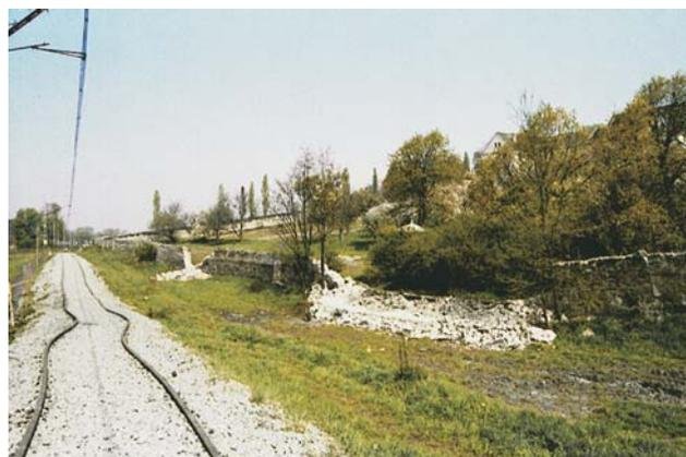
Fig. 5. Beginning of the subsiding trough formation on the outskirts of Mina crosscut. Photo by J. Przybyło
