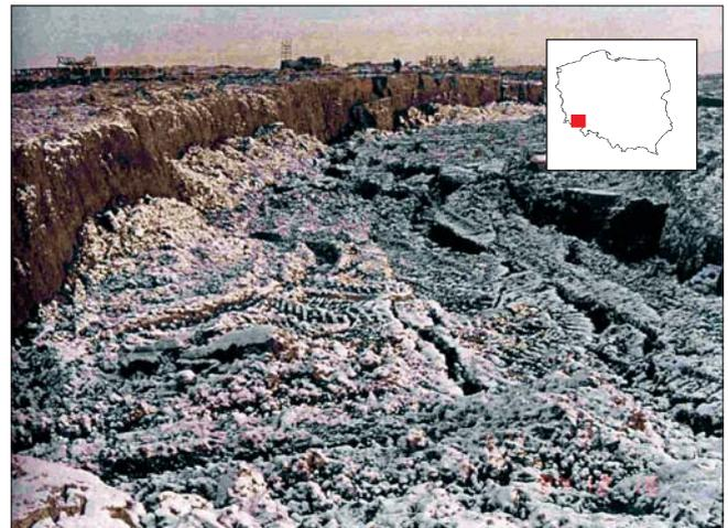
Fig. 2. Landslide on external embankments of Turów open-cast mine (6 mln m<sup>3</sup>)
