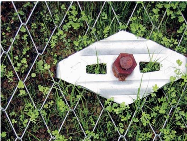
Fig. 6. High-tensile steel wire mesh TECCO
