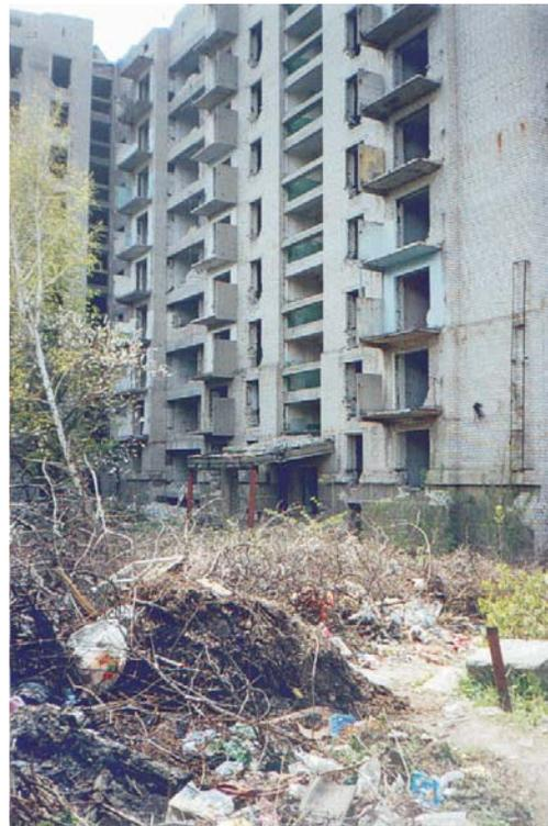
**Fig. 3. Abandon 14-storeyed dwelling house, deformed as result of landslide activation**
