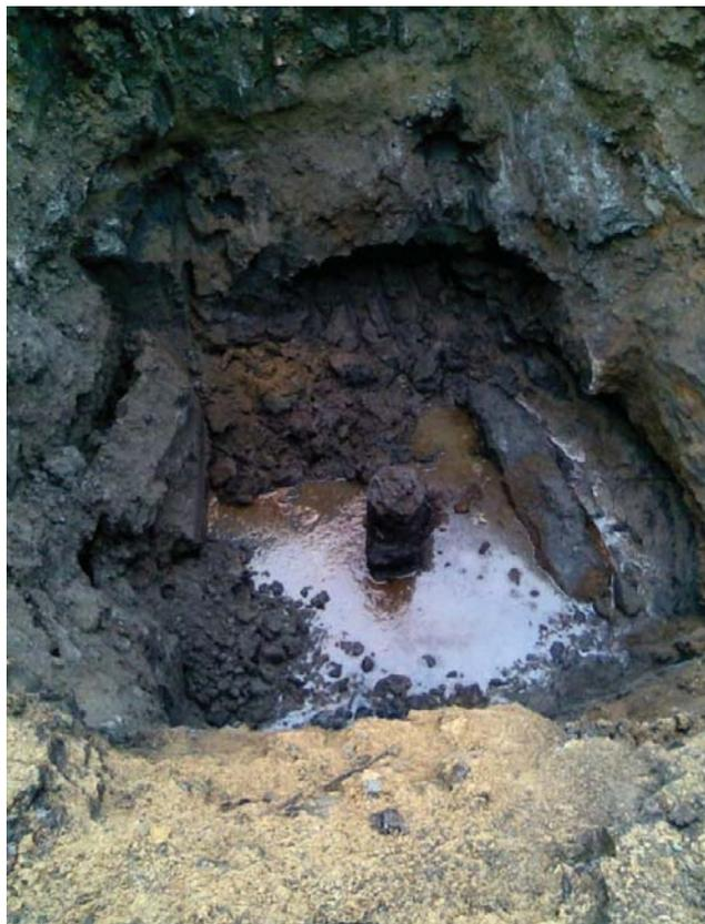
**Fig. 10.** Uncovered wellhead of the improperly abandonment HG21 well with spontaneous outflow of oil (Propagační materiál PKÚ, 2014)
