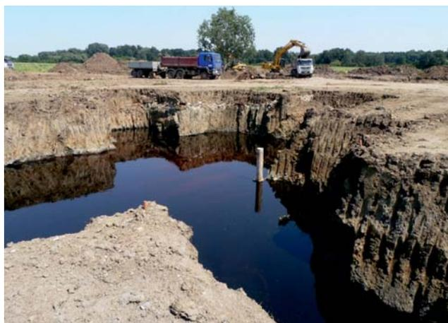
**Fig. 11.** An example of sanitation in the area surrounding the old re-abandoned wells. Contaminated soils are excavated, contaminated groundwater pumped away. Staré Pole u Nesytu (Propagační materiál PKÚ, 2014)
