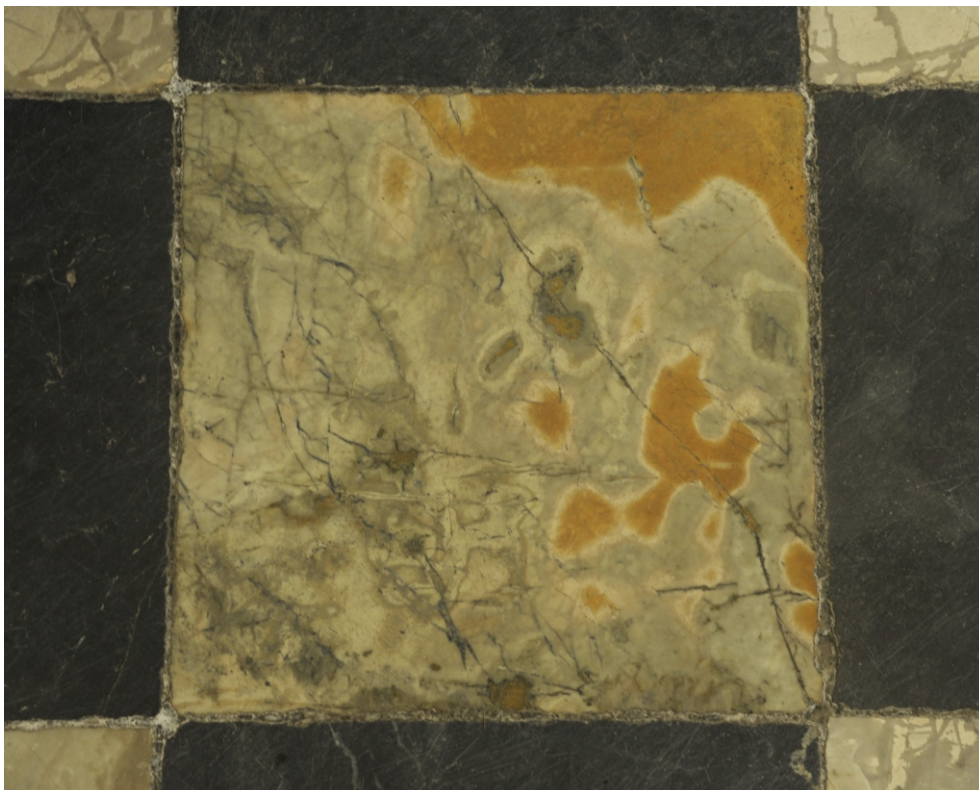
Fig. 8. Czerna, church of the Discalced Carmelites, nave, floor, “dungeon marble” tile from Dębnik, example of yellow discoloration. Dimensions: 42 x 42 cm
