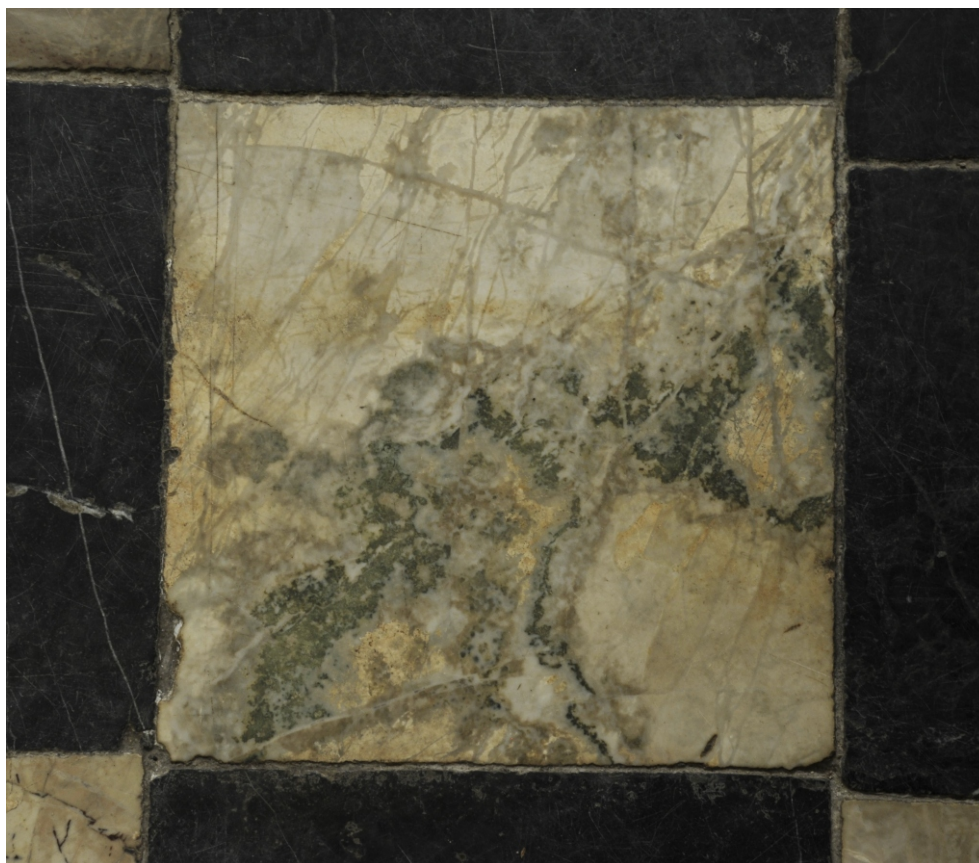
Fig. 7. Czerna, church of the Discalced Carmelites, nave, floor, after 1640–before 1690, tile made of "dungeon marble", an example of a greenish discoloration. Dimensions: 42 x 42 cm
