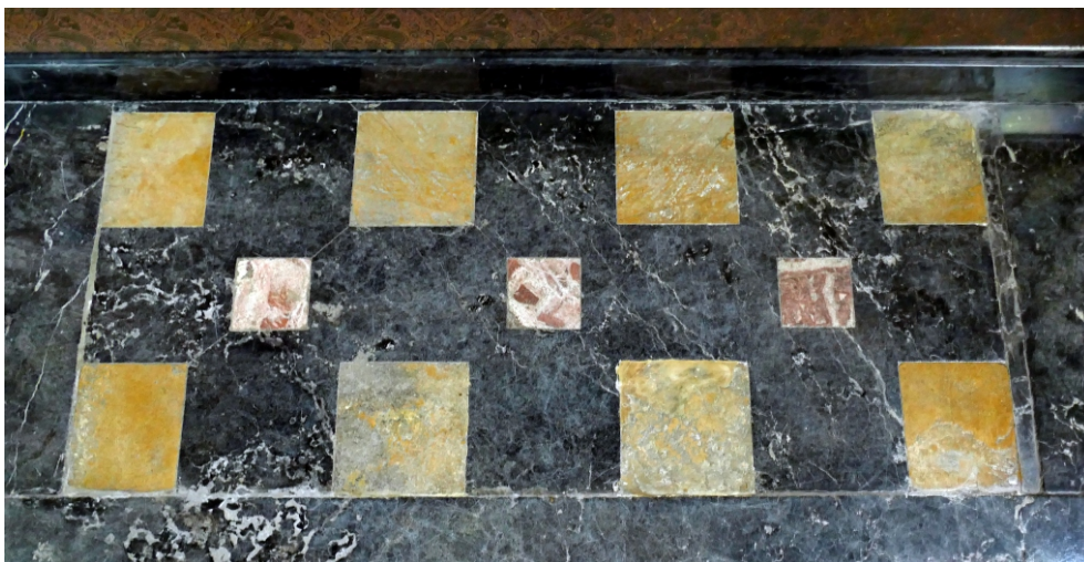
Fig. 10. Kraków-Wawel Hill, cathedral, side chapel of St. James the Apostel / Bishop Jakub Zadzik, altar step, floor, 1645–47, tiles made of "dungeon marble" from Dębnik, Dębnik limestone and vein calcite Różanka Paczółtowicka. Dimensions: 25 x 25 cm
