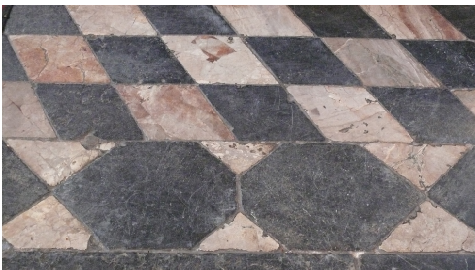
Fig. 13. Kraków, Discalced Carmelites Nuns’ church of St. Martin, “pointed” floor (today in parish church in Krzyżanowice Dolne near Pińczów on the Nida), c. 1647, “dungeon marble” tiles from Dębnik. Dimensions: 28 x 28 cm and 26 x 16 cm
