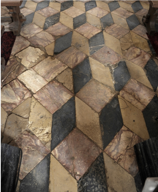
Fig. 16. Pažaislis near Kaunas, former Grand Duchy of Lithuania, church of the Camaldolese hermitage, side chapel of St. Christopher, "pointed" floor, tiles made of "dungeon marble" from Dębnik, Dębnik limestone and vein calcite Różanka Paczółtowska, around 1686, executed by Stefan Bystrzycki or Michał Poman with their studios from Dębnik. Dimensions: c. 28 x 28 cm. Photo by MW, 2013
