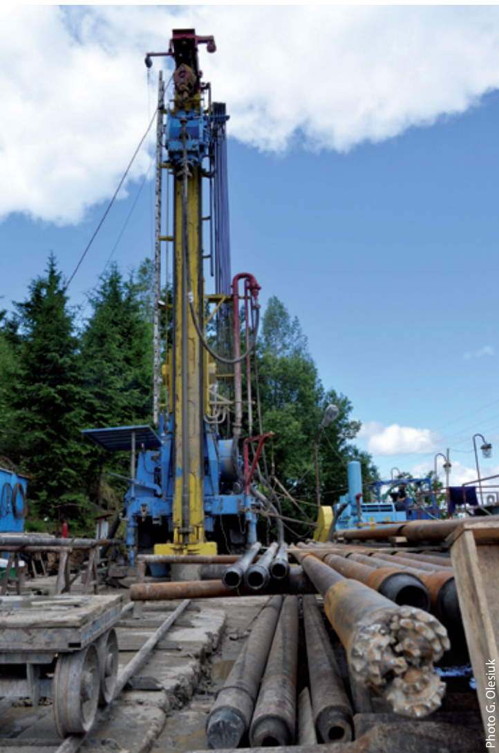
Drilling of a groundwater investigation point in Udryń, NE Poland
