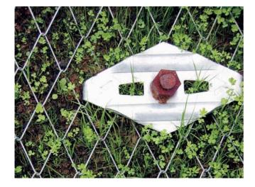
Fig. 6. High-tensile steel wire mesh TECCO
