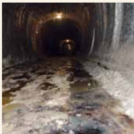
Side drift which drains effluence waters out of the landfill site
