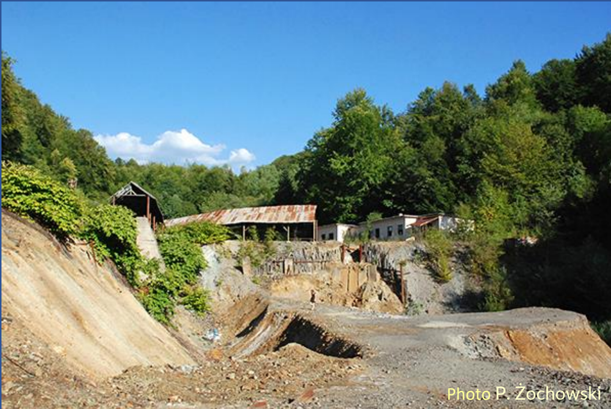
Baia Sprie old adit, 2020
