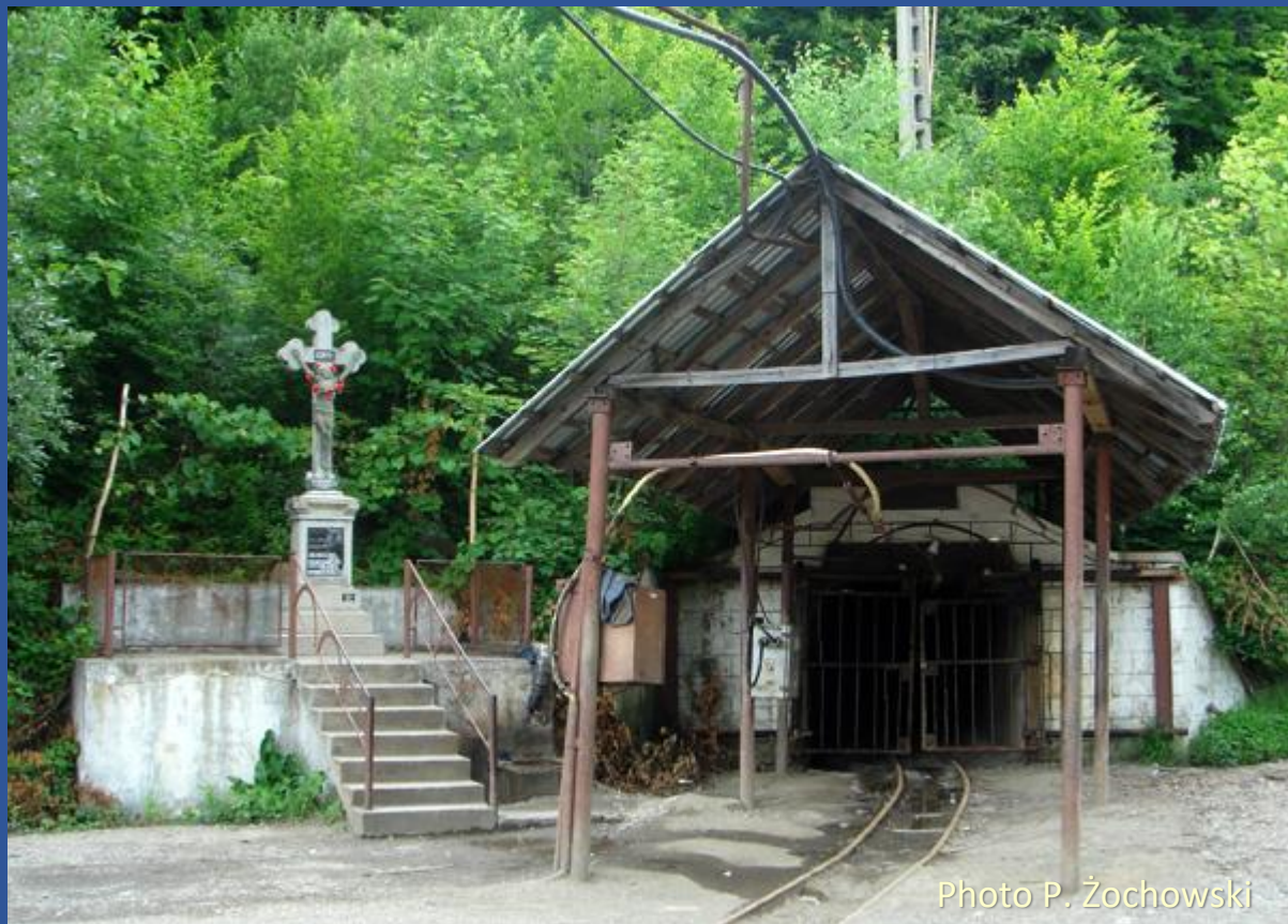
Entrance in the mine in 2005
