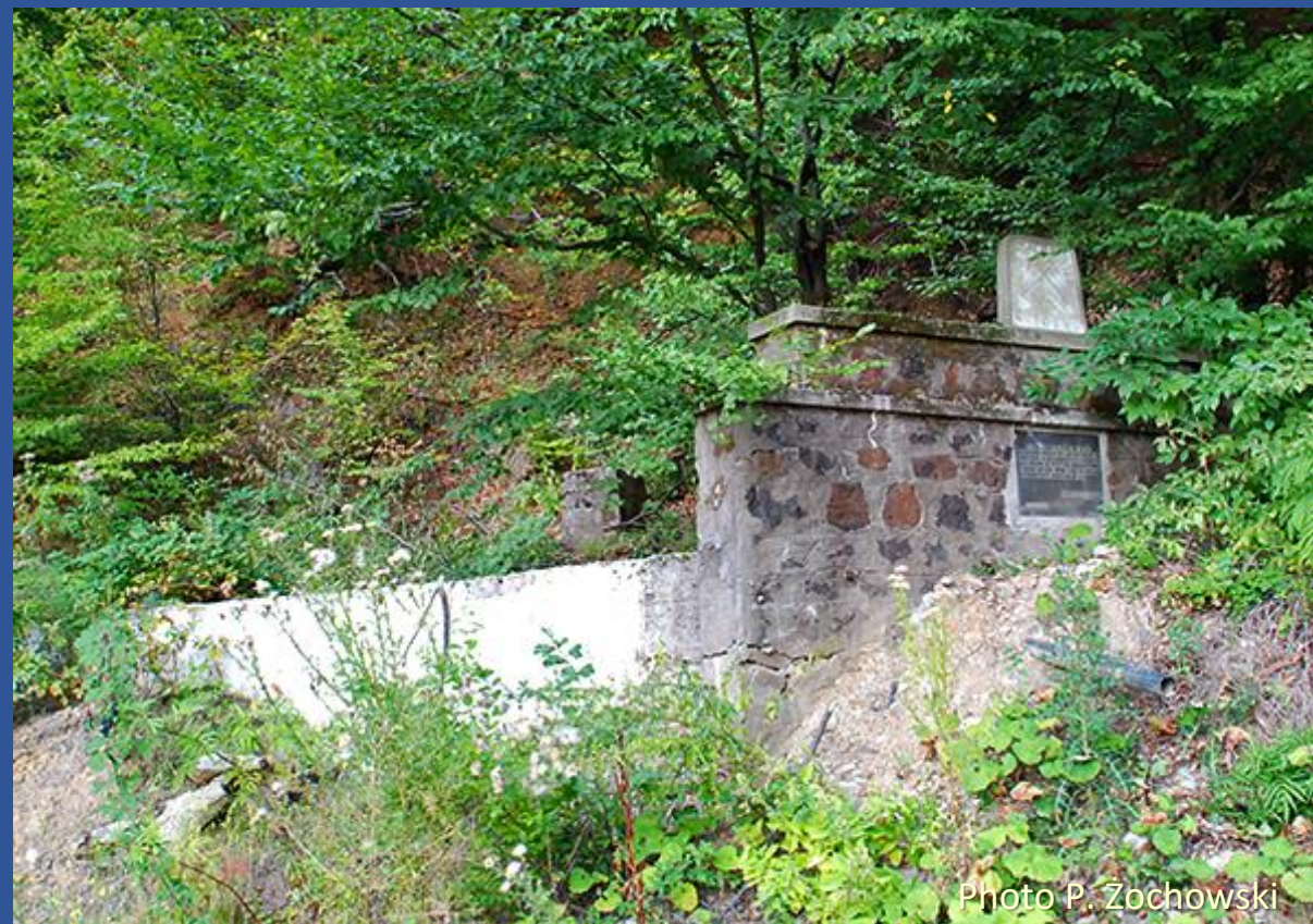
Entrance in the mine in 2020
