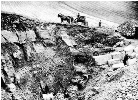
Bolechowice quarry at the beginning of XX century .– photo: Archive of the National Museum of Kielce
