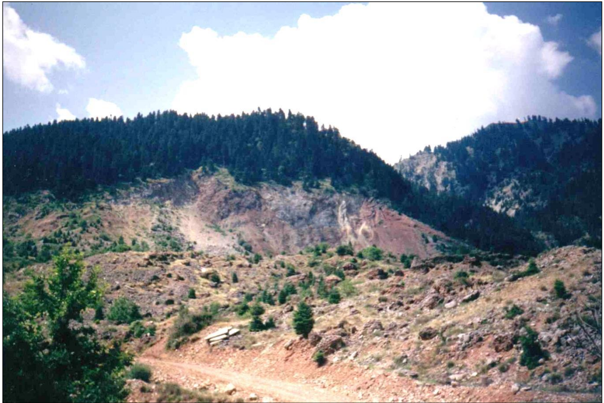
Photo 2. Landsliding masses (materials from old slides). In the background, the front of the detachment is visible.
